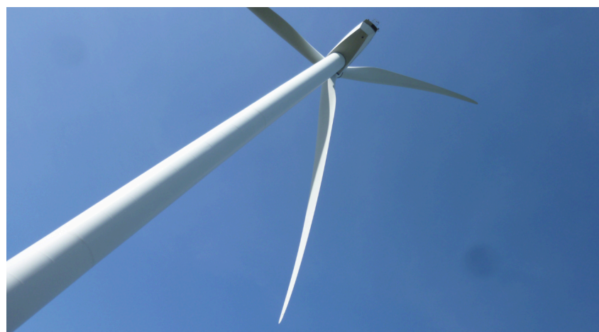
Wind turbine tower | Julieta Costa
